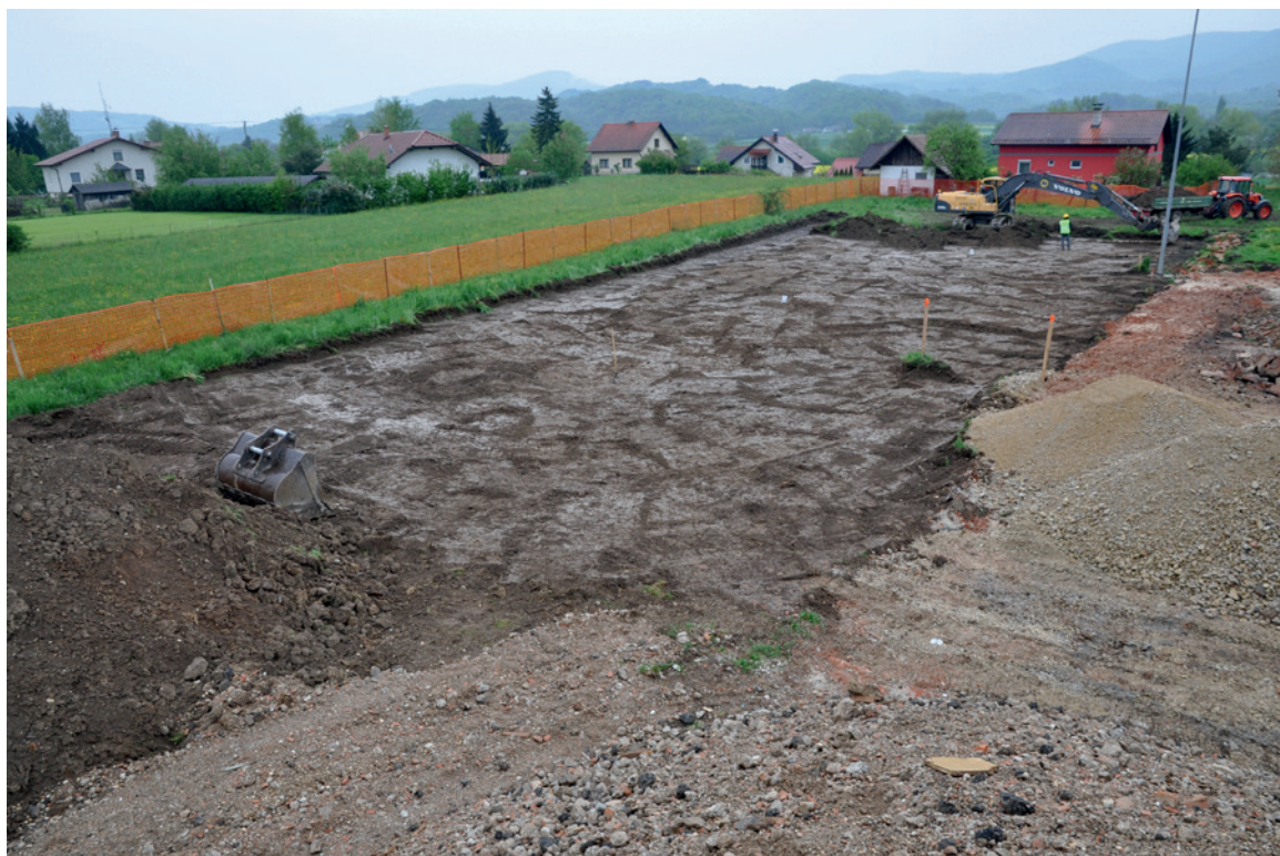
Fig. 5. View on the site at Cerklje ob Krki at the beginning of the excavation. Gorjanci hills, with well researched Late Antique hilltop settlements, are visible in the background.
