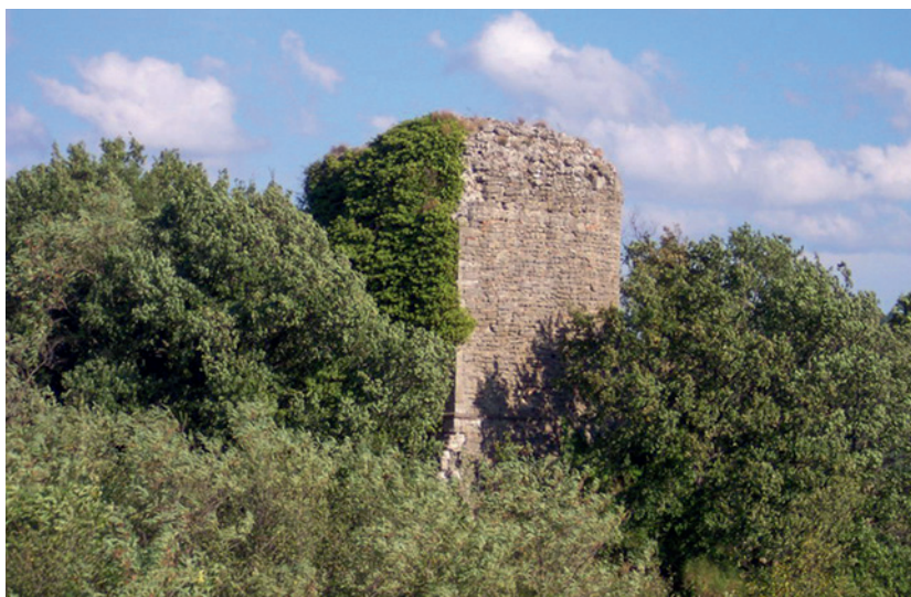
Fig. 10. The main tower of the castle of Ceparano.
